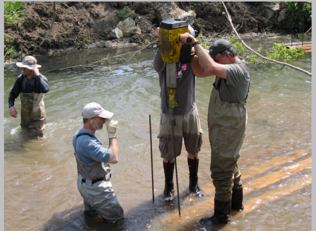
INSTALLING LUNKER STRUCTURES- PHOTO BY GREG MEYER
