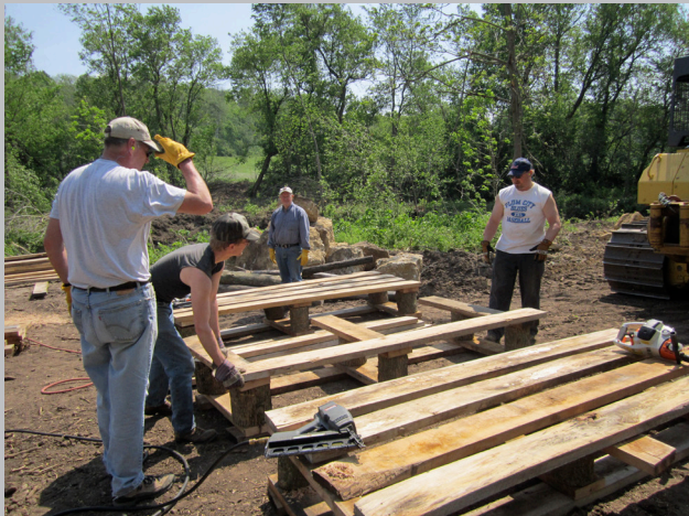
BUILDING LUNKER STRUCTURES - PHOTO BY GREG MEYER
