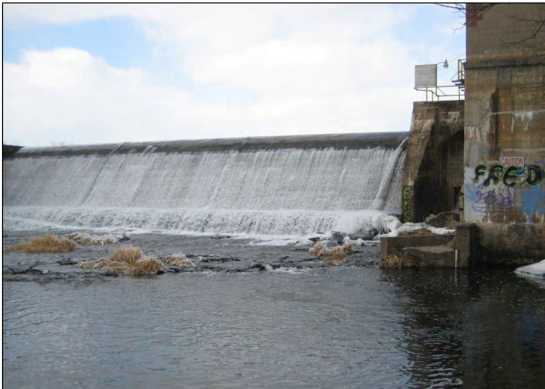
Figure 9: Existing Powell Falls Dam with power house on left bank (right of photo). The dam sits on bedrock (center of the photograph).
