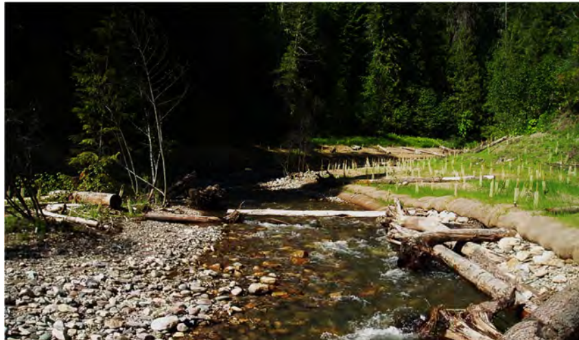
Figure 27. Cedar Creek in Ione, WA 3 months after removal of a 20ft tall dam. Over 30,000 cubic yards of sand and gravel was removed. This photo shows the restored stream channel with constructed banks, large wood habitat, pools, riffles and bars, as well as a constructed floodplain. Both planted trees and shrubs as well as naturally recruited vegetation is present.
