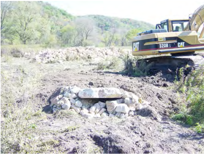
Fig. 8. Construction of a hibernaculum as part of a stream restoration project.
