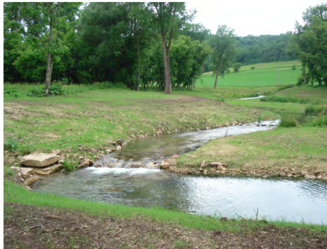
Fig. 1. Restored Driftless Area stream with armoring of the bank toe. Credit: Dauwalter.
