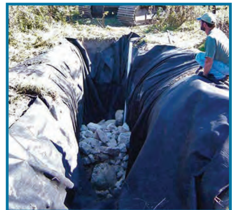
Excavate below water table one to two feet.
