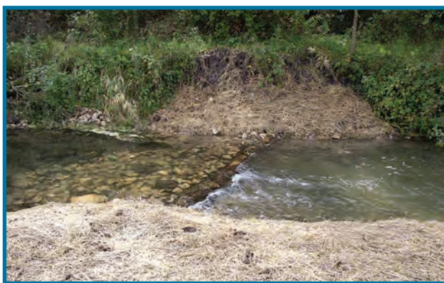
Cross channel log placed on angle to direct water flow into overhead structure.
