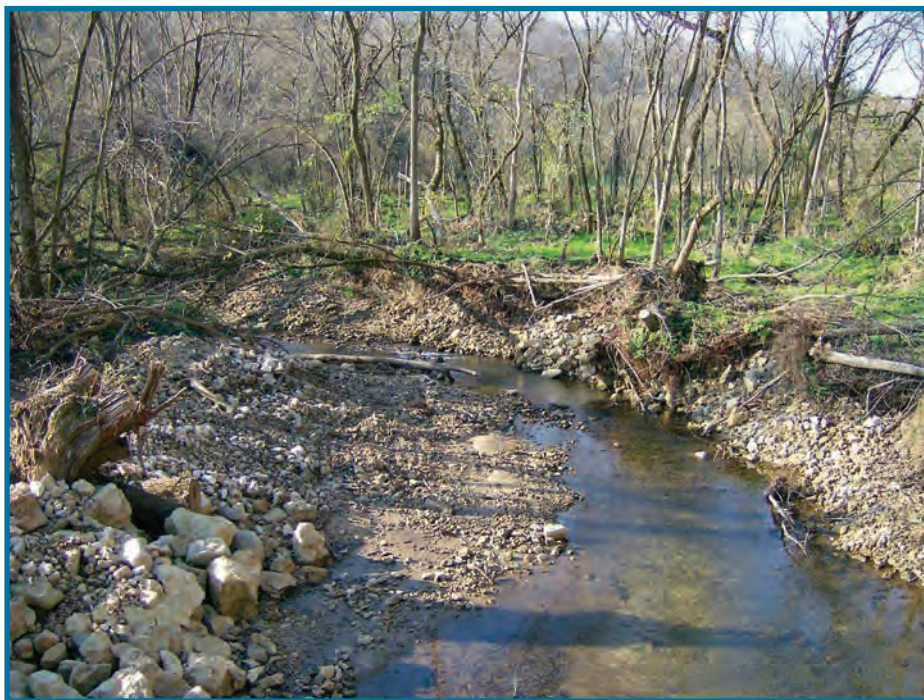
Degraded Stream in need of restoration.
