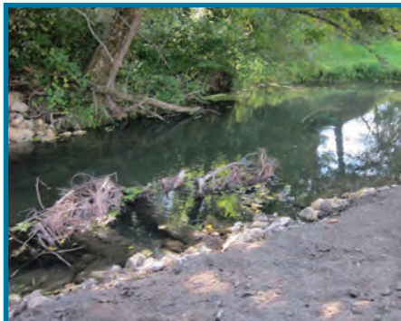
Log deflectors installed on Six Mile Branch, Iowa Co. WI
