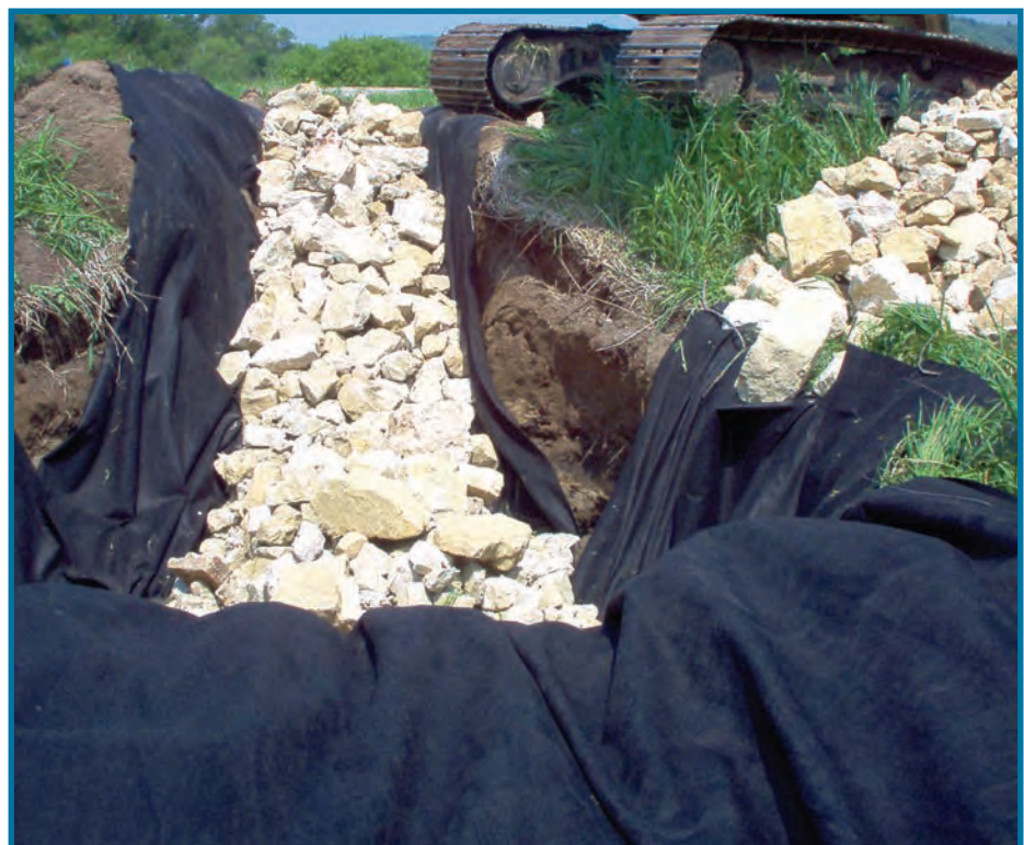
Add smaller mixed rock on top of the 8 to 10 inch bottom rock.
