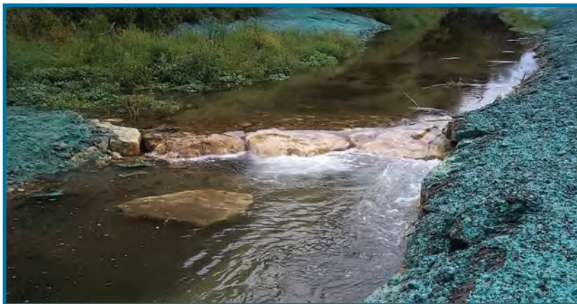
Cross channel rock weir directs water flow into skyhooks on Pine Creek, Winona, MN
