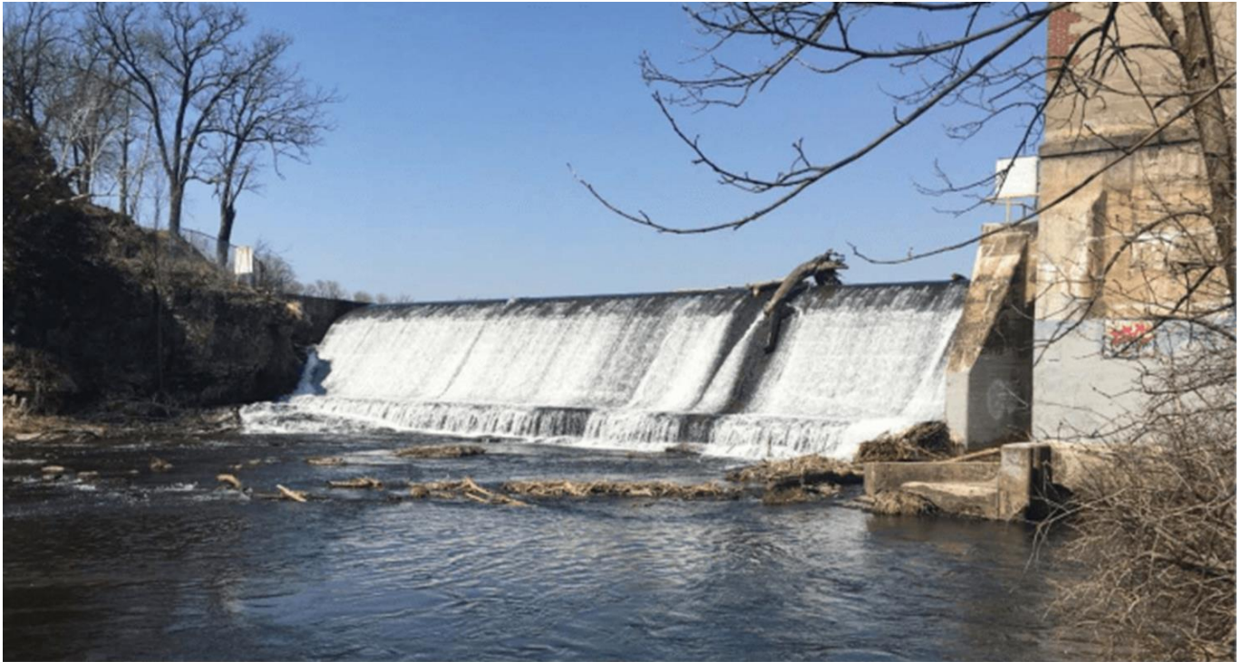
Powell Falls Dam on the Kinnickinnic River, in River Falls, WI
