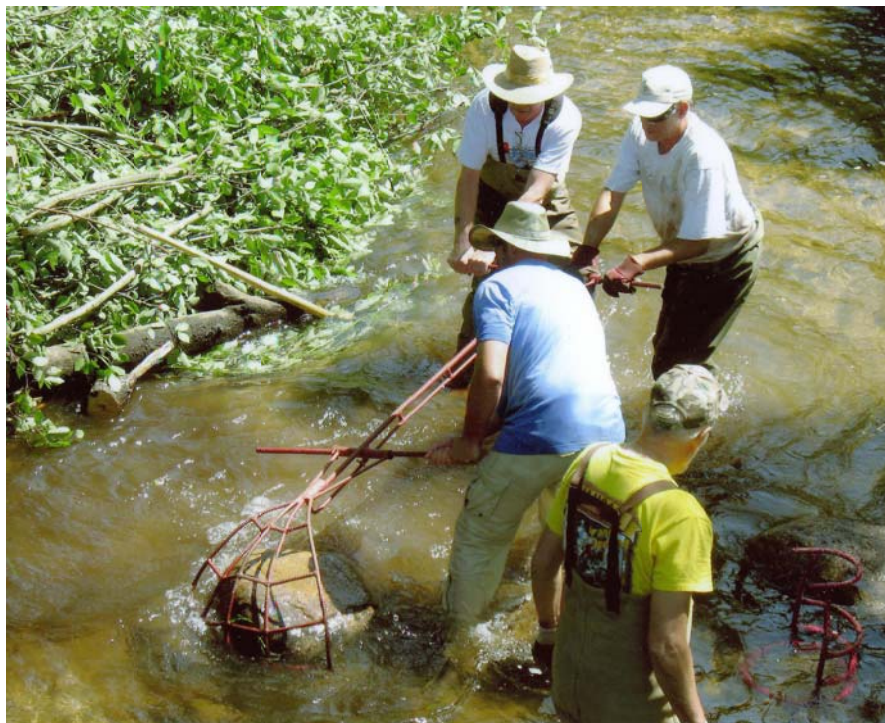
Members of the Frank Hornberg Chapter of TU using “the claw” to install boulders in the Tomorrow River
